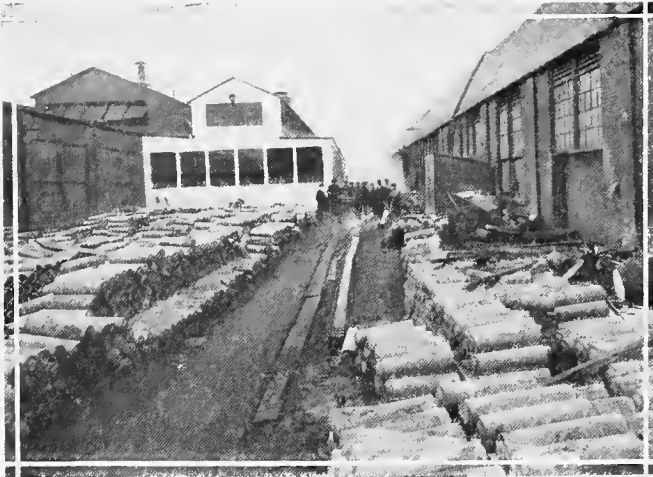
Storage of 155 mm. Shell Forgings
